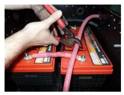
Step 4: Crimp the supplied 3/8 inch cable lugs onto the 1/0 black negative cable and the 1/0 red positive cable. Apply heat shrink to seal the connection.
