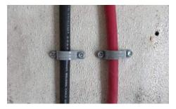
Important: Ensure that the positive and negative cables are routed so they cannot touch. Due to normal vibrations, the cables could potentially rub through the insulation, causing a short if they are touching.
