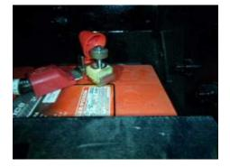
Step 13: Attach the inverter negative cable to the battery.
