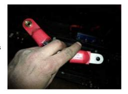
Step 12: Connect the inverter positive cable to the 150 amp fuse cube. Tighten the fuse cube nut.
