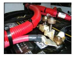
Step 12: Connect the inverter harness ground cable and the 10 gauge chassis ground cable to the negative post of the first battery.
